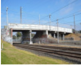
Miller Street Tramway Bridge
