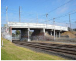
Miller Street Tramway Bridge
