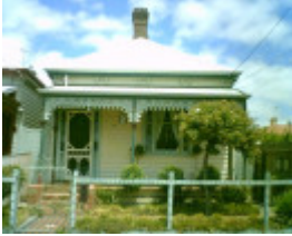
37 Lupton Street, Geelong West
