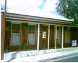
6 St James Street, Geelong West
