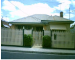
11 St James Street, Geelong West
