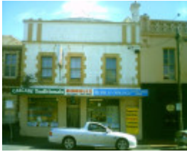
32 Aberdeen Street, Geelong West
