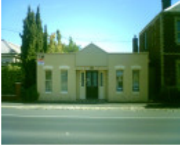
36 Aberdeen Street, Geelong West
