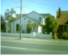
42 Aberdeen Street, Geelong West
