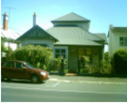
46 Aberdeen Street, Geelong West
