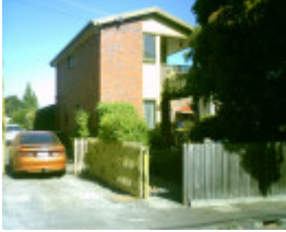
3 Emerald Street, Geelong West
