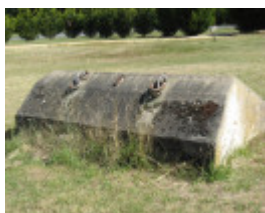
Fiskville concrete block for guy wire anchor
