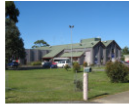
Fiskville power generating building
