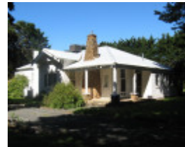
Fiskville manager's residence
