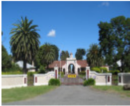
Entrance to accommodation complex
