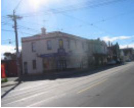
Plenty Road Commercial Precinct
