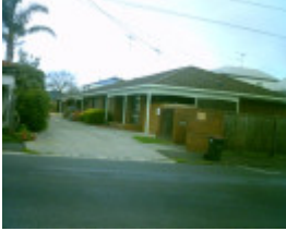
27 Candover Street, Geelong West 3 Units
