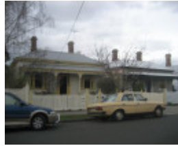
Victorian timber villas 27 and 29 Edsall Street
