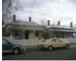
Victorian timber villas 27 and 29 Edsall Street
