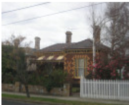
Victorian polychrome brick villa at 12 Parkside Street
