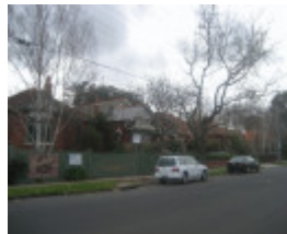
Edwardian villas on the west side of Thanet Street
