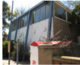
Former Shire Offices_Benalla_front_KJ_5/9/08
