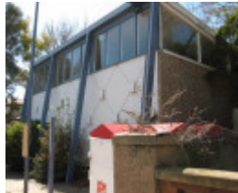
Former Shire Offices_Benalla_front_KJ_5/9/08
