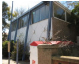
Former Shire Offices_Benalla_front_KJ_5/9/08
