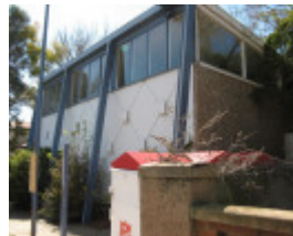
Former Shire Offices_Benalla_front_KJ_5/9/08
