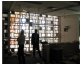
Former Shire Offices_Benalla_screen from inside_KJ_Sept 08
