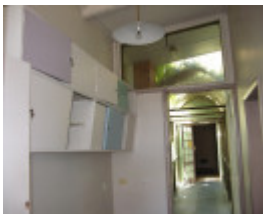
Former Benalla Shire Offices_kitchen cupboards_KJ_Sept 08
