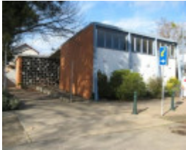
Former Shire Offices_Benalla_JC_Aug 08
