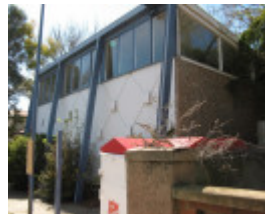
Former Shire Offices_Benalla_front_KJ_5/9/08
