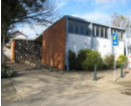
Former Shire Offices_Benalla_JC_Aug 08
