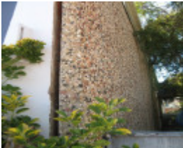
Former Shire Offices_Benalla_aggregate wall_KJ_5/9/08
