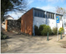
Former Shire Offices_Benalla_JC_Aug 08
