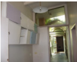
Former Benalla Shire Offices_kitchen cupboards_KJ_Sept 08
