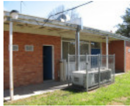
Former Benalla Shire Offices_rear wall_KJ_Sept 08
