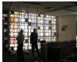
Former Shire Offices_Benalla_screen from inside_KJ_Sept 08
