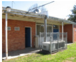
Former Benalla Shire Offices_rear wall_KJ_Sept 08
