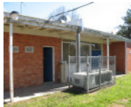
Former Benalla Shire Offices_rear wall_KJ_Sept 08
