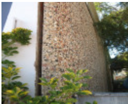
Former Shire Offices_Benalla_aggregate wall_KJ_5/9/08
