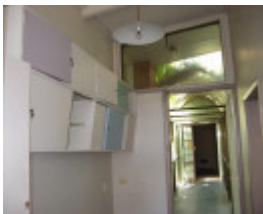
Former Benalla Shire Offices_kitchen cupboards_KJ_Sept 08
