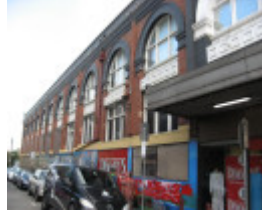
Dimmeys_Richmond_Green St elevation_9 July 08
