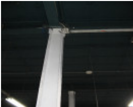
Dimmeys_Richmondinterior columns_9 July 08
