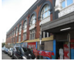
Dimmeys_Richmond_Green St elevation_9 July 08
