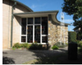
45050 St Faiths Anglican Church Glen Iris exterior of former baptistry 2010
