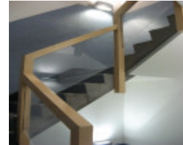
Plumbers & gasfitters stairwell
