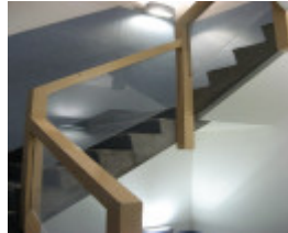
Plumbers & gasfitters stairwell
