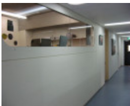
Plumbers & gasfitters ground floor corridor
