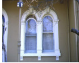
barcelona terrace brunswick steret fitzroy window detail
