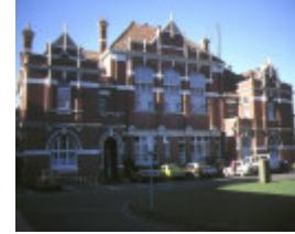
1 ballarat high school sturt street west ballarat front view apr1987
