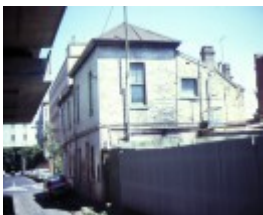
former devonshire arms hotel fitzroy street fitzroy rear view feb1982
