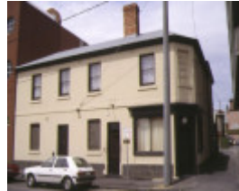
1 former devonshire arms hotel fitzroy street fitzroy front view feb1982
