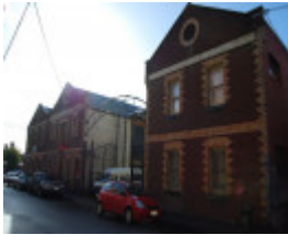
4555 Former Cordial Factory View North East 10
