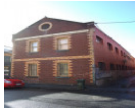
4555 Former Cordial Factory 10
