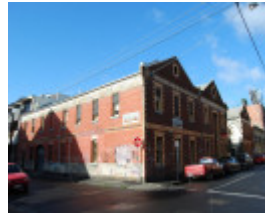
4555 Former Cordial Factory View South East 10
