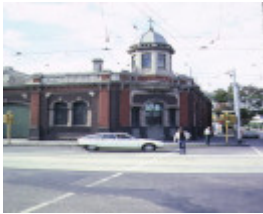
1 cable tram engine house gertrude street fitzroy front corner tower jan1983
