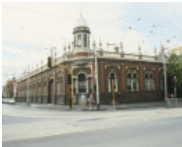
cable tram engine house gertrude street fitzroy street view
