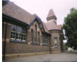
1 primary school 773 caulfield south window detail
