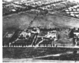
45841 McKay Housing Estate - King Edward Ave
