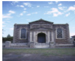
Former Wesleyan Church Parsonage & Common School James Street Port Fairy Front View of Church February 1990
