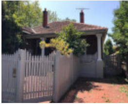
73 Stanhope Street, Malvern
