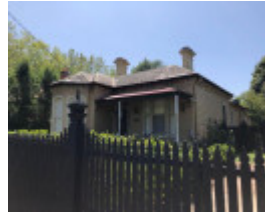
75 Stanhope Street, Malvern
