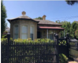
75 Stanhope Street, Malvern
