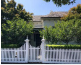
81 Stanhope Street, Malvern
