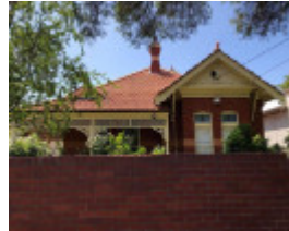
83 Stanhope Street, Malvern
