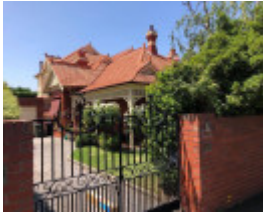
83 Stanhope Street, Malvern
