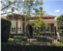
87 Stanhope Street, Malvern
