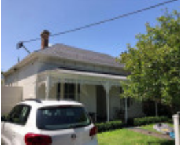
89 Stanhope Street, Malvern
