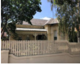
91 Stanhope Street, Malvern
