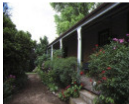
millbank grant street bacchus marsh verandah
