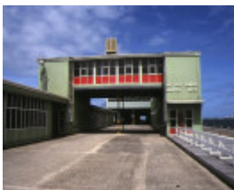
station pier port melbourne port workers amenities block
