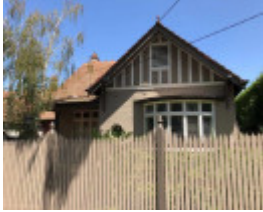
80 Stanhope Street, Malvern
