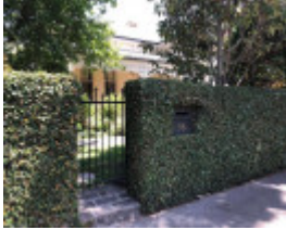
96 Stanhope Street, Malvern
