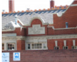
PRIMARY SCHOOL NO. 734 SOHE 2008
