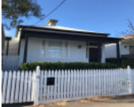
32 Westbourne Street, Prahran
