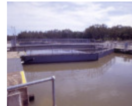
h00993 torrumbarry weir lock chamber steam boiler and steam winch complex torrumbarry lock stream upstream gates she project 2004
