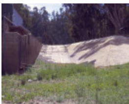
h00993 torrumbarry weir lock chamber steam boiler and steam winch complex torrumbarry trestle runway ramp she project 2004
