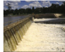
1 torrumbarry weir complex face of weir
