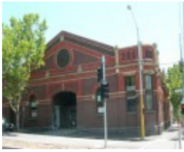
FORMER CABLE TRAM ENGINE HOUSE AND CABLE TRAM TRACK FORMATION SOHE 2008
