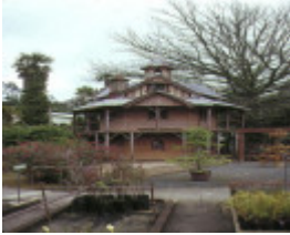
1 state nursery office creswick front view sep1989
