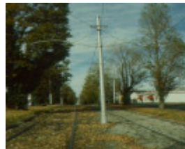
ornamental tramway overhead poles peel street
