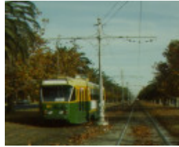
1 ornamental tramway overhead poles dandenong road
