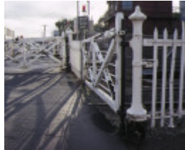
1 interlocked railway crossing gates anderson street yarraville closed interlocked gates apr1994
