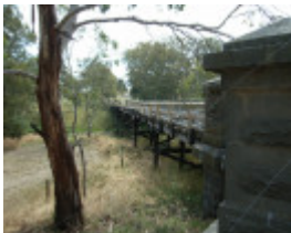
ELLERSLIE BRIDGE SOHE 2008
