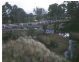
1 ellerslie bridge over hopkins river ellerslie side elevation
