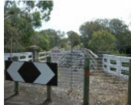
ELLERSLIE BRIDGE SOHE 2008
