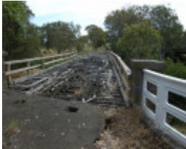
ELLERSLIE BRIDGE SOHE 2008
