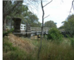
ELLERSLIE BRIDGE SOHE 2008
