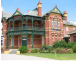
BUNDOORA PARK HOMESTEAD SOHE 2008
