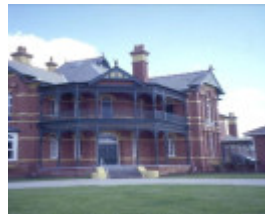
bundoor homestead snake gully drive bundoor facade she project 2003
