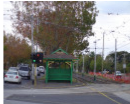
H0230 Tram shelter Dandenong Rd Caulfield May 2006 side view pj
