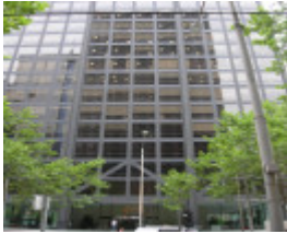
FORMER BHP HOUSE SOHE 2008
