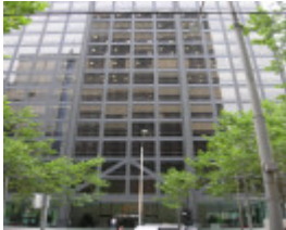
FORMER BHP HOUSE SOHE 2008
