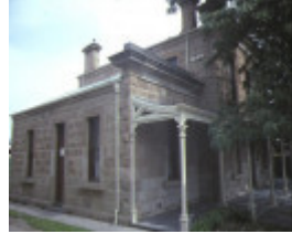
bacchus marsh court house main street bacchus marsh verandah view sep1984
