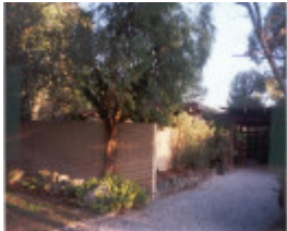
47068 House - 3 Exford Close, Donvale
