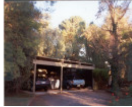
47068 House - 2 Exford Close, Donvale
